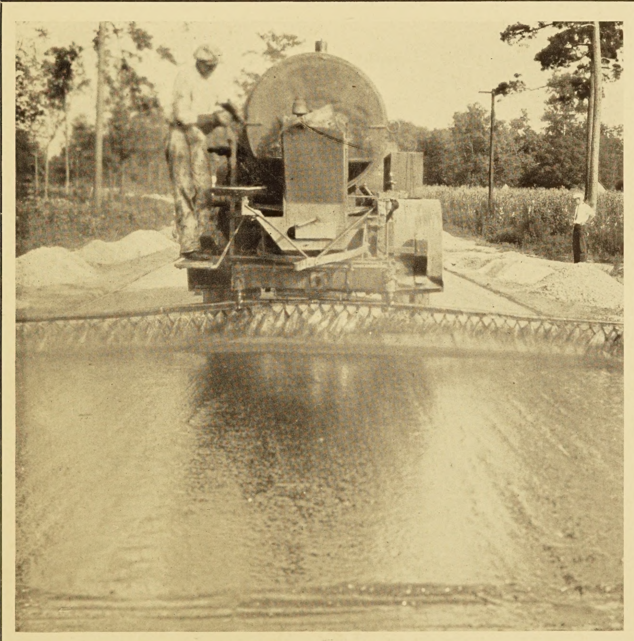
APPLYING PRIME COAT TO SAND-CLAY BASE
